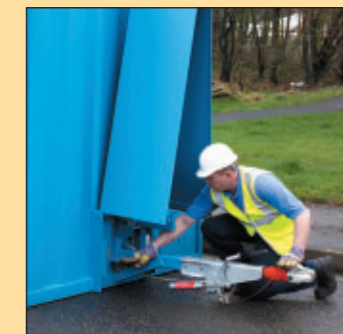
2 minutes: Hydraulics lowers unit to ground
